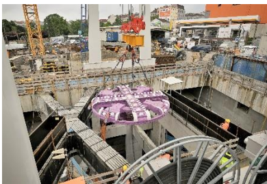
The cutting wheel, the centrepiece of the TBM, at Matzleinsdorfer Platz. It weighs approx. 78 tonnes, has a diameter of 6.88 metres and is equipped with around 40 rolling chisels and 100 peeling knives. © ARGE U2 17-21
