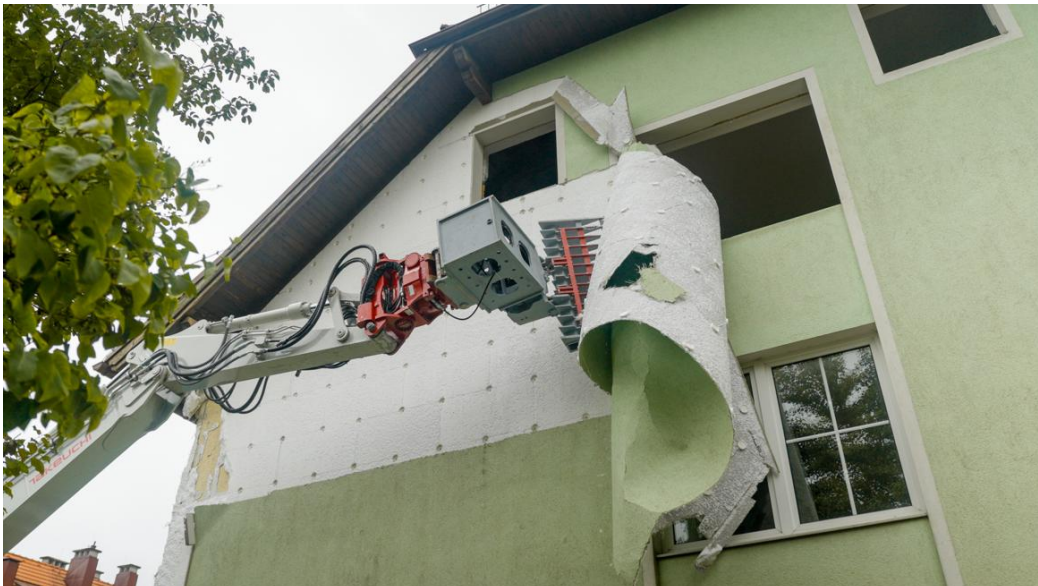
Excavator attachment in action: The PORR team is able to remove residual materials from the EPS during the demolition process itself © ORBIS Development
