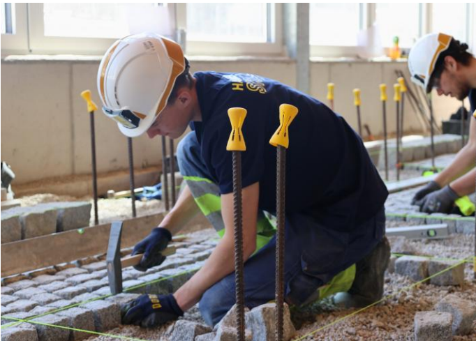
The civil engineering task involved paving © PORR
