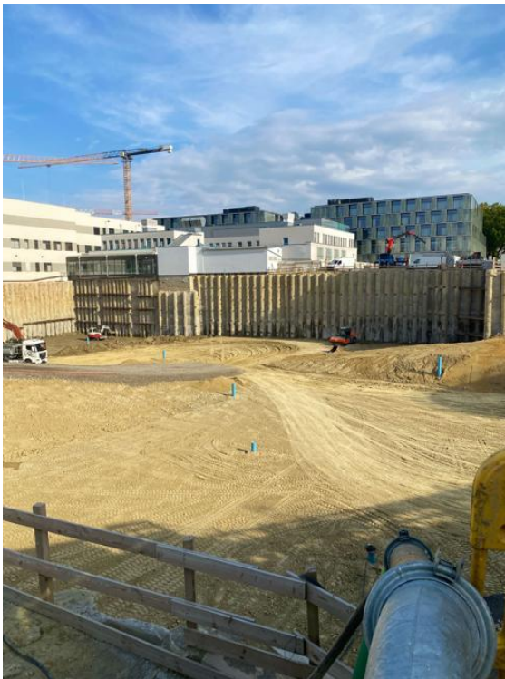
10,500 m 2 excavation pit for the new central emergency department at Klinik Favoriten © PORR
