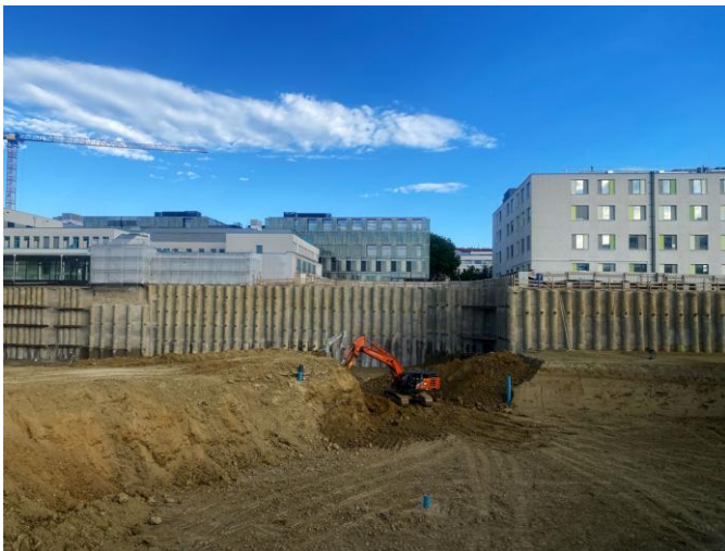
By the end of August, 14,275 tonnes of clay-rich material had been recovered from the pit © PORR
