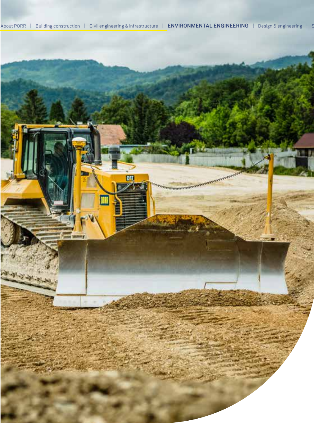
Flood retention basin Fahrafeld/Lower Austria – Austria Earthworks at the largest retention basin in Lower Austria
